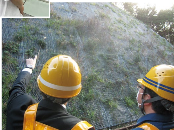
(Rockfall prevention work)
